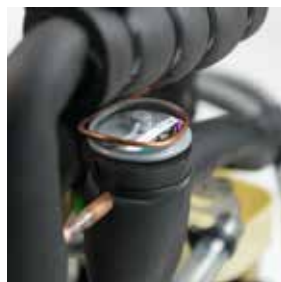
Thermal expansion valve increases performance for all conditions.
